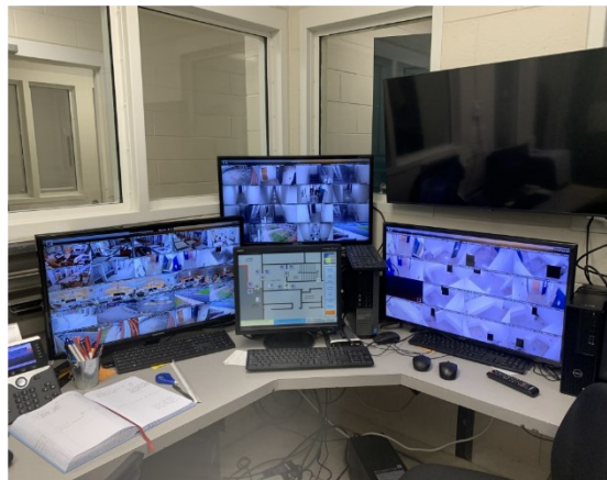
Security Control Room
