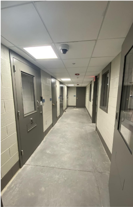
Secure Holding Corridor
