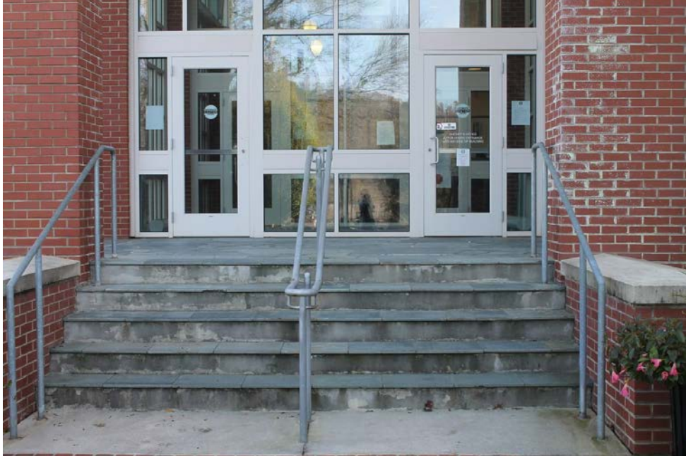
Main Courthouse Entry
